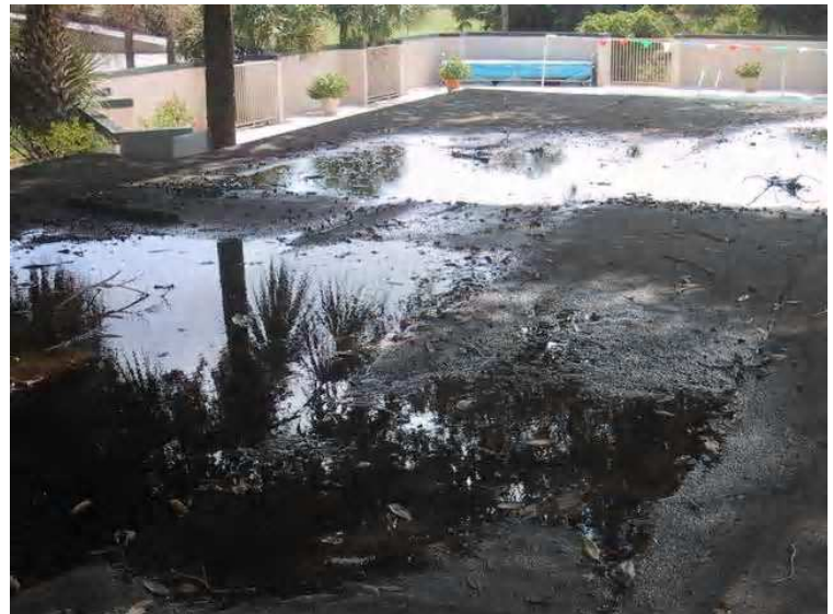
Fitness Center Roof - Shows low spot where water is pooling, note growth of mold-like substances.
